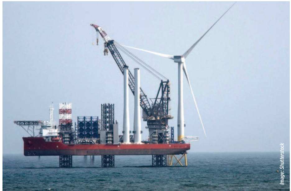
The largest wind farm installation vessel in the world and the first turbine installed off the coast of Aberdeen. Balmedie, Aberdeenshire, Scotland, UK. April 11th 2018.
