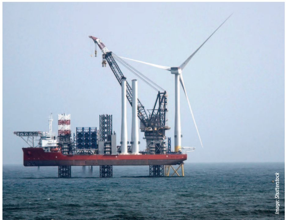
The largest wind farm installation vessel in the world and the first turbine installed off the coast of Aberdeen. Balmedie, Aberdeenshire, Scotland, UK. April 11th 2018.
