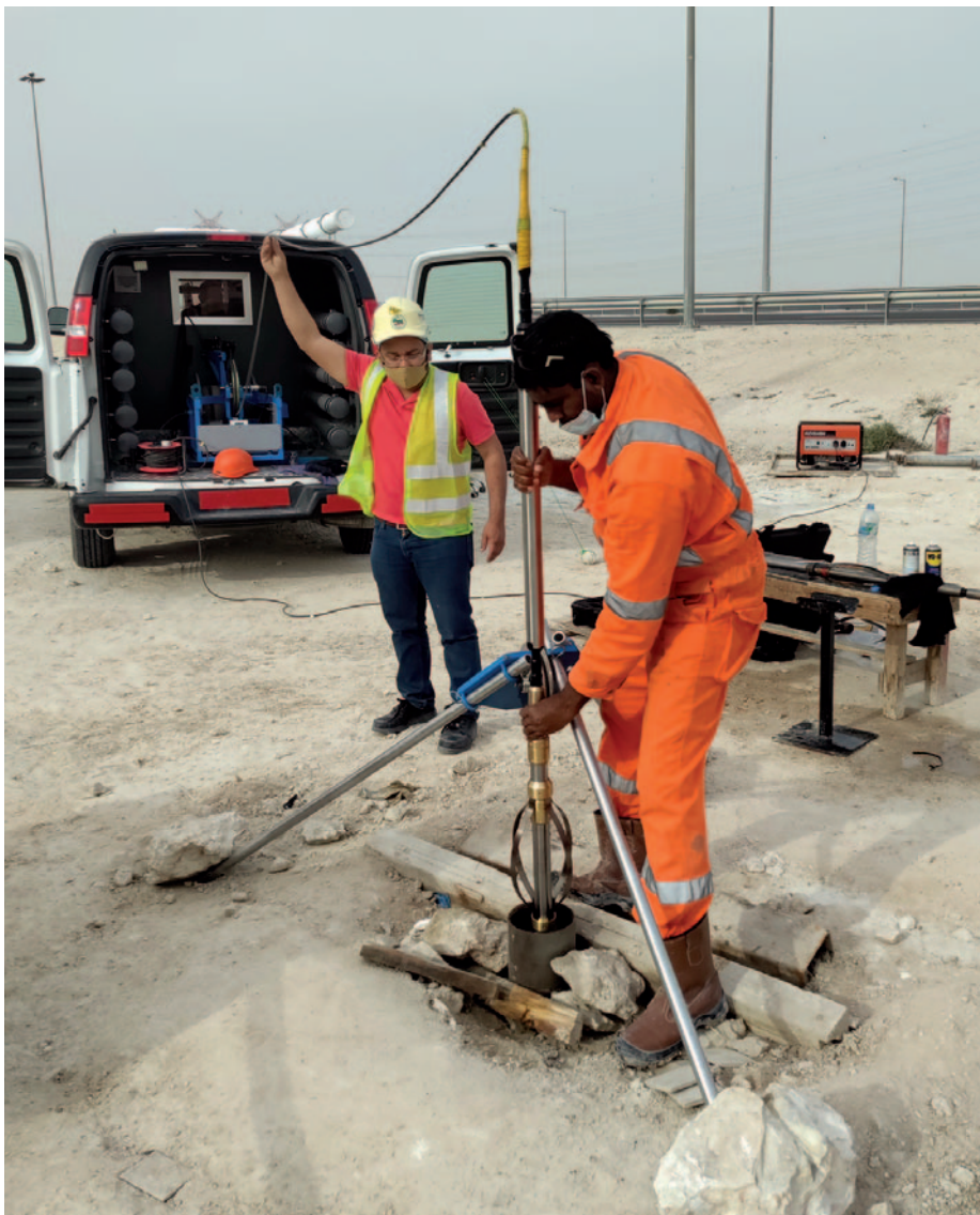
RGeo-eye® downhole camera with sinker bar applied to the geotechnical borehole.
