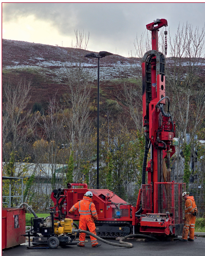
Rotary core drilling at Tre Morfa.
