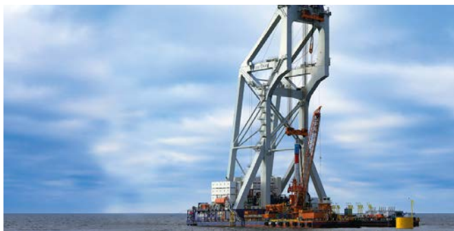
Van Oord's recently upgraded heavy lift installation vessel Svanen at work at the Baltic Power offshore wind farm
