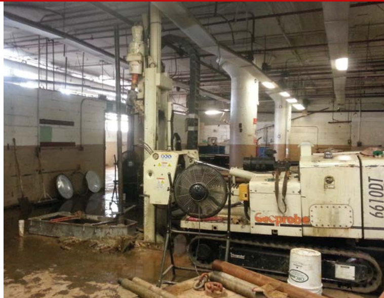
When clearance falls below 15ft, specialised, low-clearance drill rigs with short towers are employed by Aquifer Drilling & Testing
