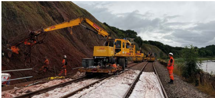
Rockfall netting being installed with rock bolts along the Severn Estuary line to help prevent further line closures due to slope failures
