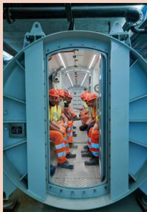
Trained workers enter the hyperbaric regime for the Casalnuovo tunnel project through gradual adaptation in a special compensation chamber
