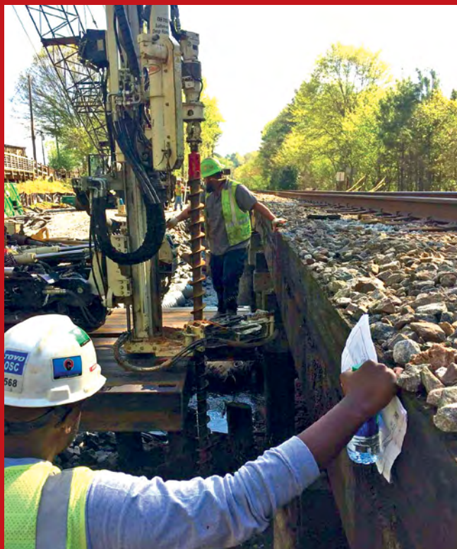
Dangling auger rods 25ft next to a train trestle to complete Geotech SPT and rock coring with Geo Lab Drilling’s Geoprobe 7822DT
